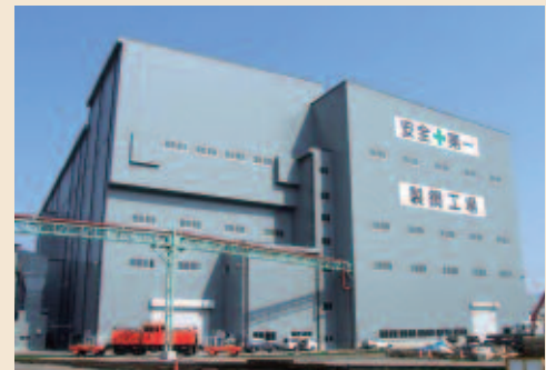
The facility at our Muroran Plant currently undergoing expansion (Steel ingot production plant)
