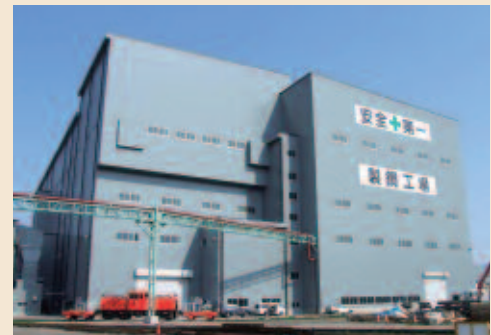
The facility at our Muroran Plant currently undergoing expansion (Steel ingot production plant)
