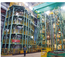
熱処理炉 Heat Treatment Furnace
